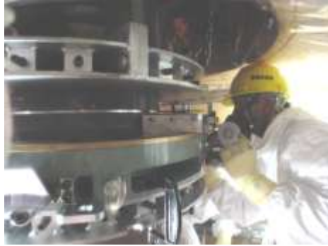
Cut off the Outer Piping
