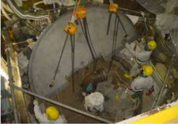
Remove Radiation Shielding Plate
